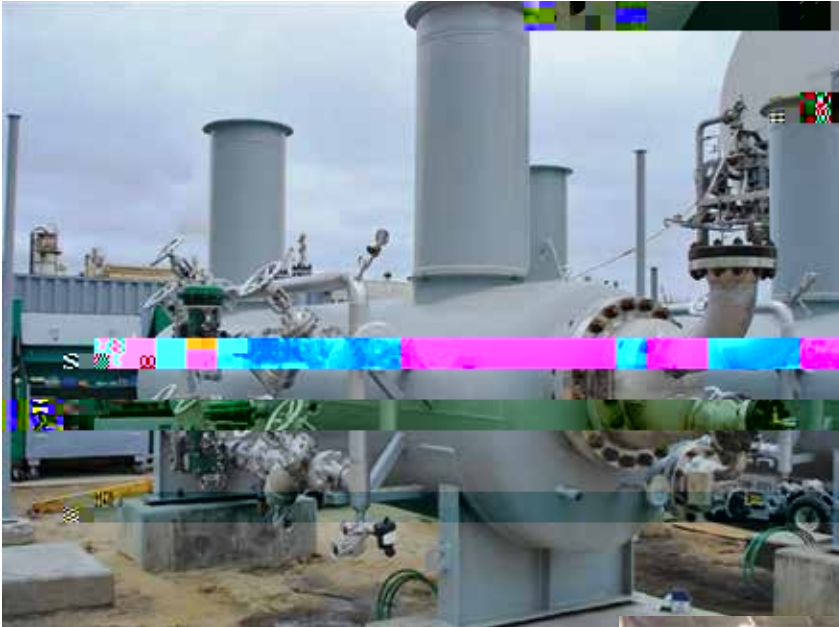
Compact Configuration with Process and Pressure-Building Bundles
